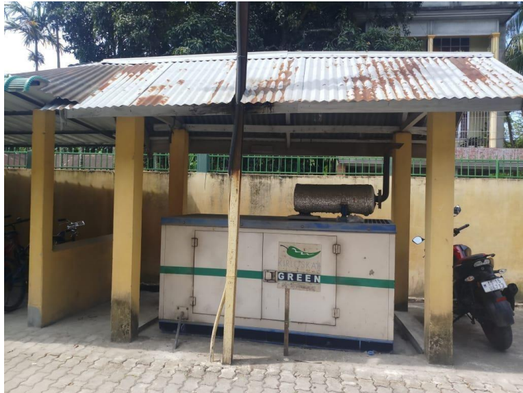
Figure 3: Diesel Generator (DG)
