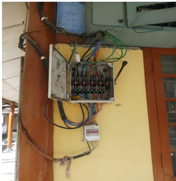
Figure 10: Alternating current obtained from Roof Top Solar Plant is directly interfaced with APDCL supply contributing to energy demand of the college during daytime/solar generation period and thereby reducing overall consumption from APDCL.
