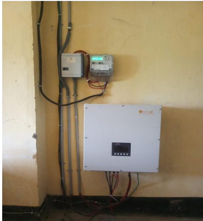
Figure 9: Solar Inverter system for interfacing of ON-GRID 20kWp Solar Roof Top system with APDCL mains. DC generated from solar panels converted to AC for usage.
